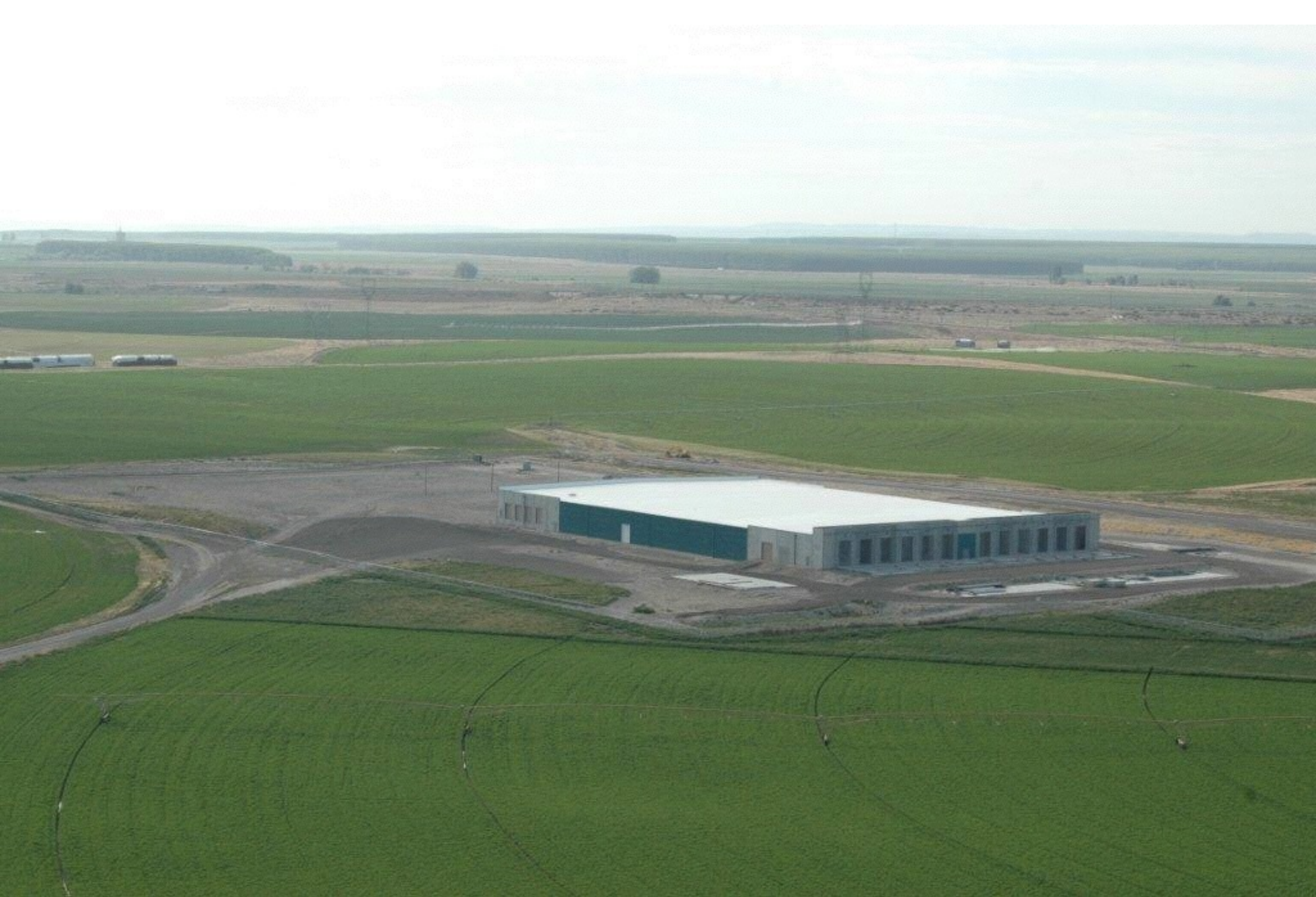
Amazon Data Center, 2012
